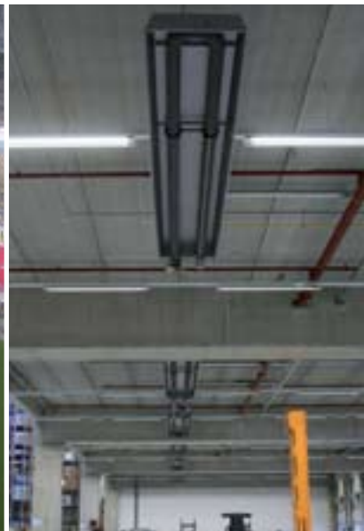
Heating of logistics halls with low-intensity heaters
